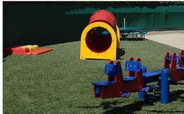
Synthetic Playground Grass Installation in Santa Monica, California.
